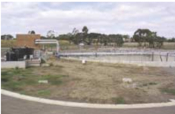
Colac wastewater reclamation plant
