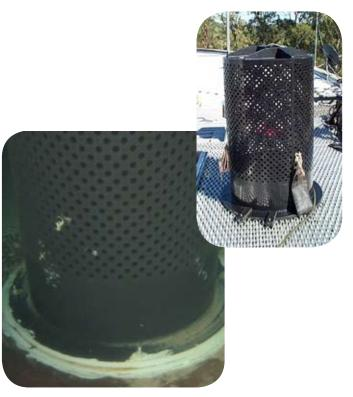
the uneven concrete surface. The screen was fitted by divers using an airpowered drill to place 16mm SS tru-bolts through the base flange and into the concrete floor. The tru-bolts were dipped in NMP 1720 epoxy to seal them into the concrete and avoid future 'Crevice corrosion'. The base flange area was also sealed to the floor using 1720 epoxy with good results.
