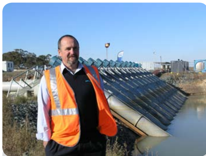
Jim Wheelhouse - Project Manager, Goulburn-Murray Water at the Major Pumping Station pump suction inlet.
