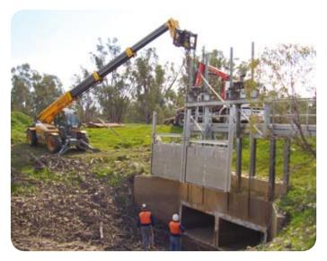
New gates and guides were designed by AWMA to ensure acceptable actuator operation and reduced maintenance. The new gates consist of aluminium reinforced plate undershots with aluminium guides. The reinforced gates are a fraction of the weight of the existing mild steel gates and run in low friction HDPE (high density polyethylene) guides.
