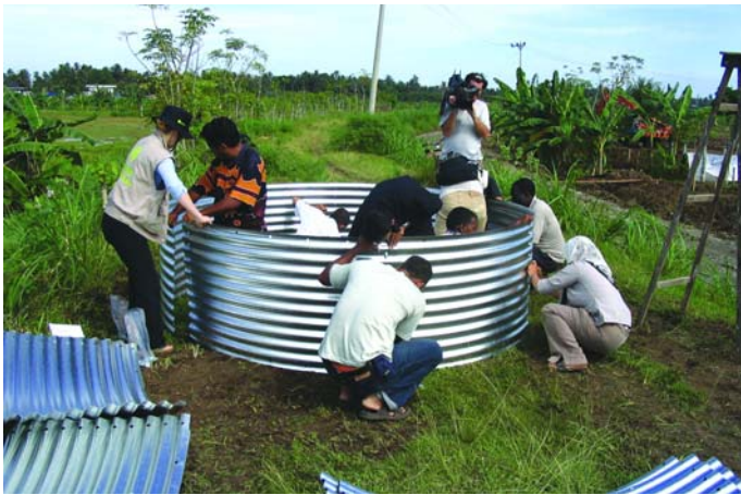
Constructing water tanks Below The finished product
