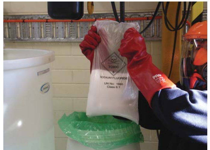
Loading 5kg bags of Sodium Fluoride into the saturation tank
