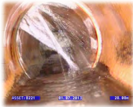
Figures 4 & 5: Photos Showing Heavy Infiltration before and after Relining
