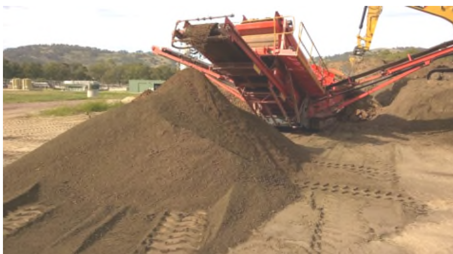
Figure 2: Screen used for the Biosolids and Sand Blending Process
