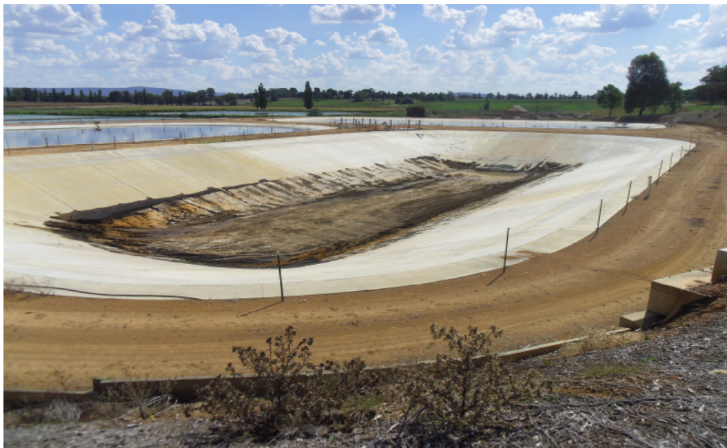
Figure 1: Emptied Lagoon Sand Filter and Underdrainage Removed
