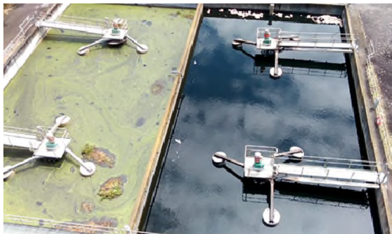
Figure 2: Tanilba Bay WWTW IDEA / Sludge Lagoon Arrangement
