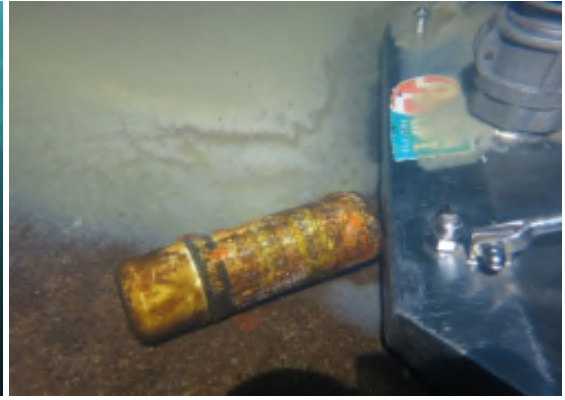
Figure 8: Excessive Sediment and Debris
