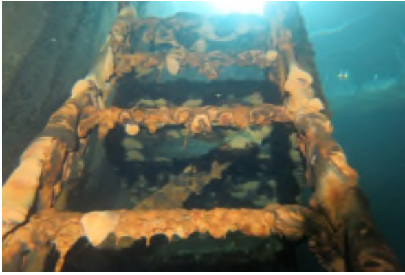
Figure 7: Corroded Ladder
