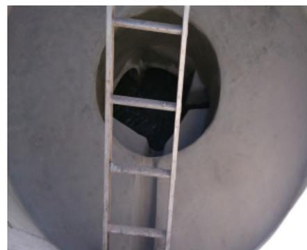
**Figures 1 & 2:** *The receiving manhole was cut off above pipe level using a diamond rope saw. Six screw piles sunk to a depth of 6 metres were used to take the weight of the above concrete chamber which formed the temporary well.*
