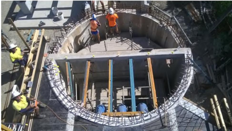
**Figure 9:** *Forming the lid over the well and discharge valve pit*
