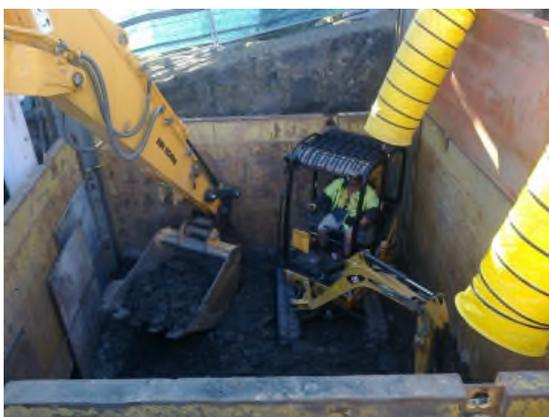
**Figure 4:** *Excavators digging pit*
