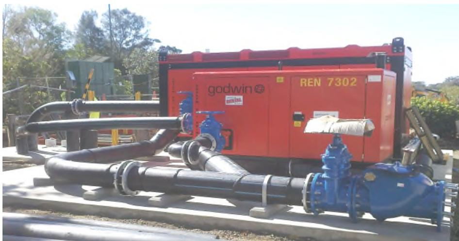
**Figure 3:** *Using the new well and the existing retic system as storage, the diesel pumps were capable of diverting the flow around the well, pumping at a maximum rate of 170 L/sec.*
