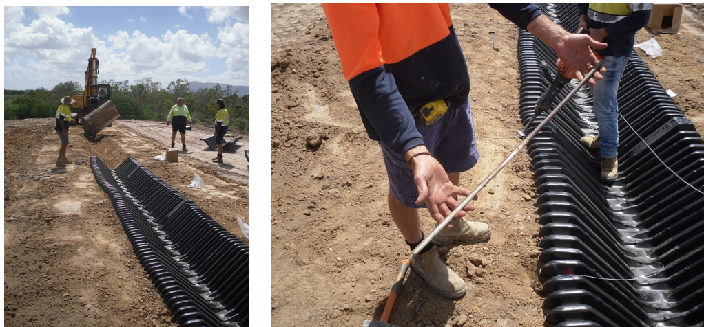
Figure 3: Trench Excavation and SmartDitch® Installation
