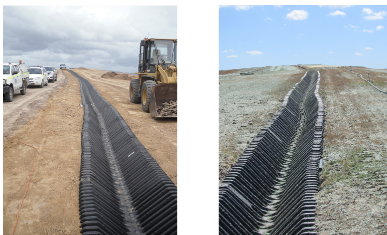
Figure 4: SmartDitch® Installation
