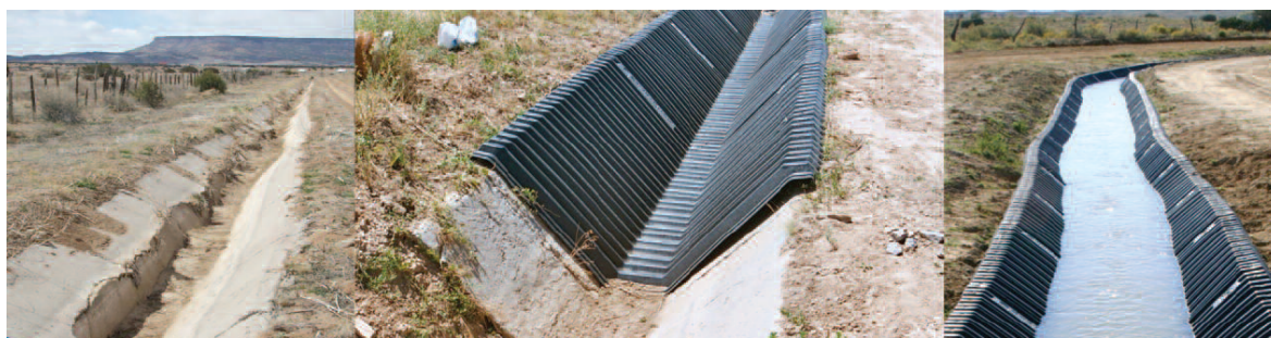
Figure 2: Before, During and After Photos of the First SmartDitch® Installation
