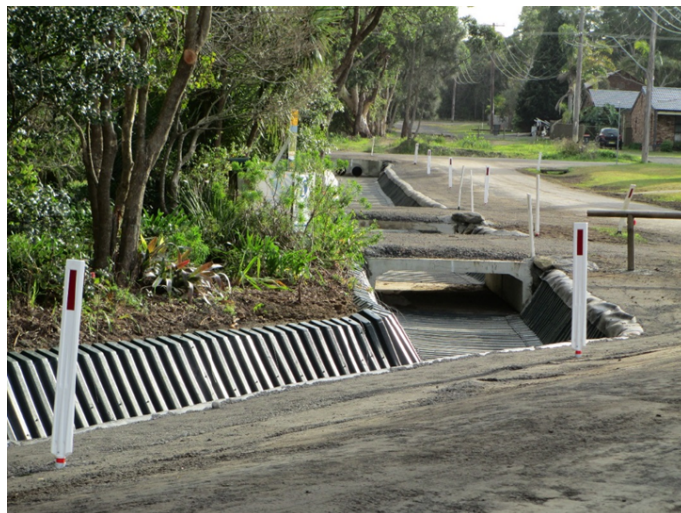
Figure 7: Box Culvert Residential Property Accesses
