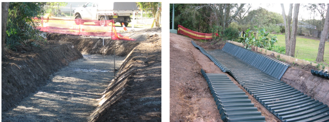
Figure 6: Construction of the Megaditch Channel
