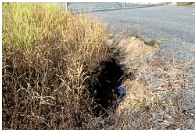
Figure 1: Examples of Eroded Open Channels
