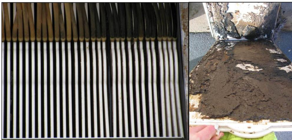
**Figure 1:** *Sludge caking between membrane sheets (Te Aroha 24/05/2010) causing displacement of neighbouring sheets*
