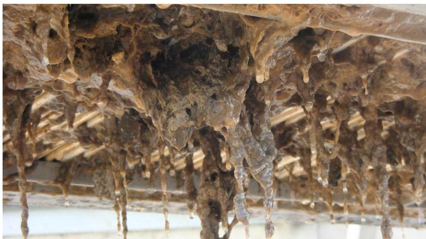
***Figure 2:*** *Example of lint/hair agglomeration under membrane module (Turangi WWTP)*
