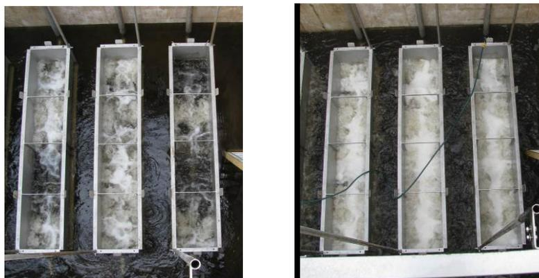
***Figure 3: Coarse Bubble Aeration Pattern Pre Diffuser Cleaning (left) and Post Diffuser Cleaning (right) [Te Aroha WWTP]***
