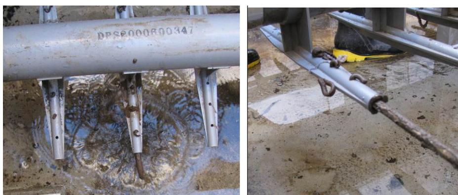
***Figure 4: Coarse bubble aeration diffuser cleaning [Te Aroha WWTP]***
