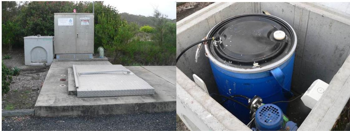
**Figure 1:** Typical MgOH installation at Sewage Pump Station
