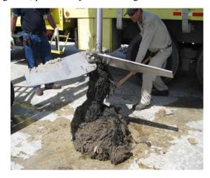
Figure 2: Clearing the impeller
