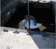
Figures 4 & 5: The first Clean-Edge impeller installed in STP in USA
