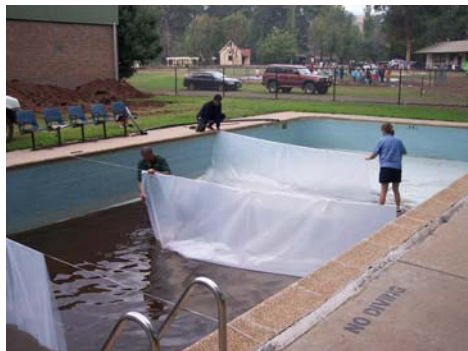
Figure 5: Temporary baffles in the Licola swimming pool
